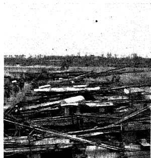
A pontoon bridge across the Grand Canal near Taierchwang, constructed by the Chinese of canal boats. In the background may be observed some of the Chinese dugouts which dotted the northern bank.
